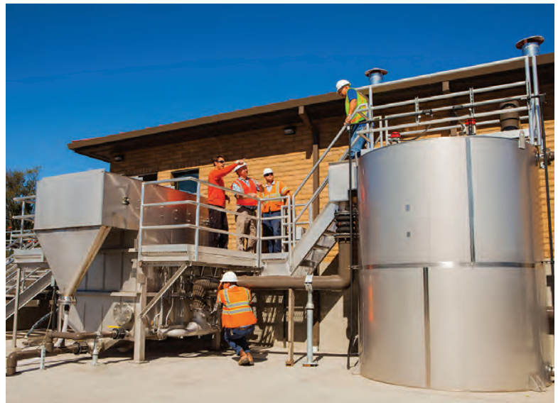
The Suspended Air Flotation (SAF) system from Heron Innovators has one-tenth the connected hp and one-fifth the footprint of conventional approaches. It also uses less chemistry while generating substantially higher percent algae solids.
