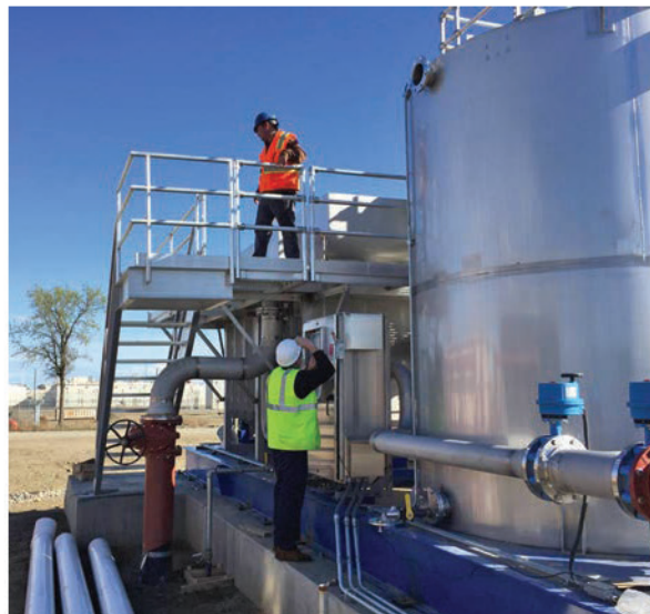
The Suspended Air Flotation process was used with dual-media filtration to produce the Title 22 reuse water.
